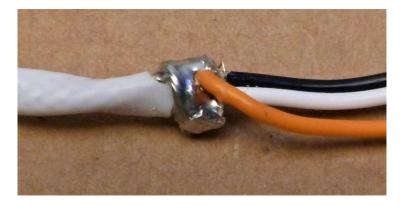
Cover the soldered connection with heat shrink tubing.
